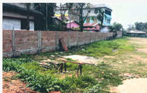
Boundary Wall, The Scholar School, Guwahati
