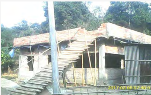
Community Centre at Hailakandi, Lalamukth, Assam (South)
