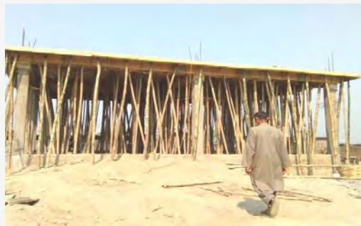
Community Centre at Barpathar, Morigaon District, Assam (North)
