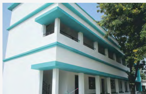
Newly constructed Building with 8 Class rooms
