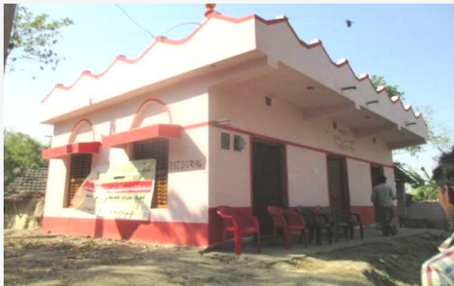
Community Centre at Milangarh, Malda West Bengal. Capacity: 80
