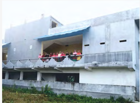
West Bengal: Hostel Building, Annajath Hostel, Sahabajpur, Charka Tola, kaliachak, Malda, W. B - Building with 4 rooms
