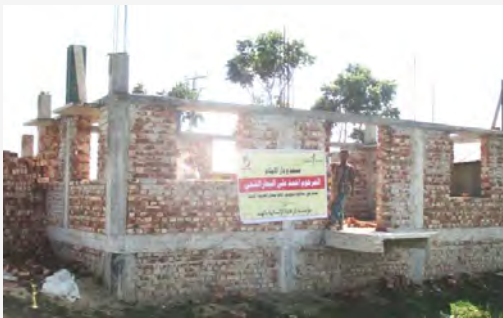
Community Centre: Joharpur, Dinajpur District, West Bengal
