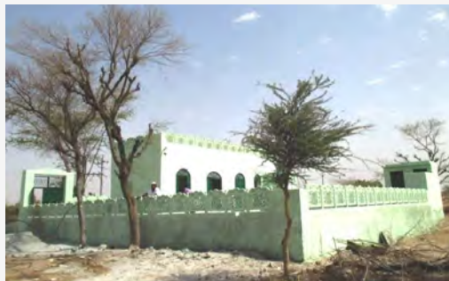
Community Centre at Panneki Badia, Bijaynagar, Ajmer, Rajasthan. Boundary wall and Tube well are also Constructed.
